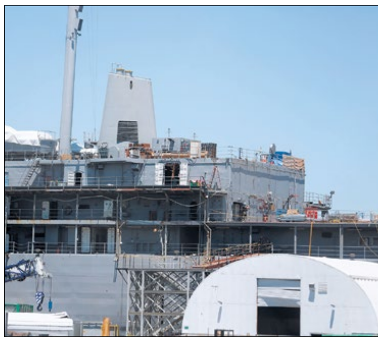
The USS Emory S. Land is undergoing scheduled maintenance to the deck, turbines, heating, ventilation and air conditioning systems at Mare Island, Calif. The ship is shown July 11.
